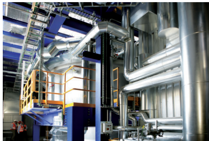
Fluidized bed incinerator for thermal treatment of oil shale at a cement plant
